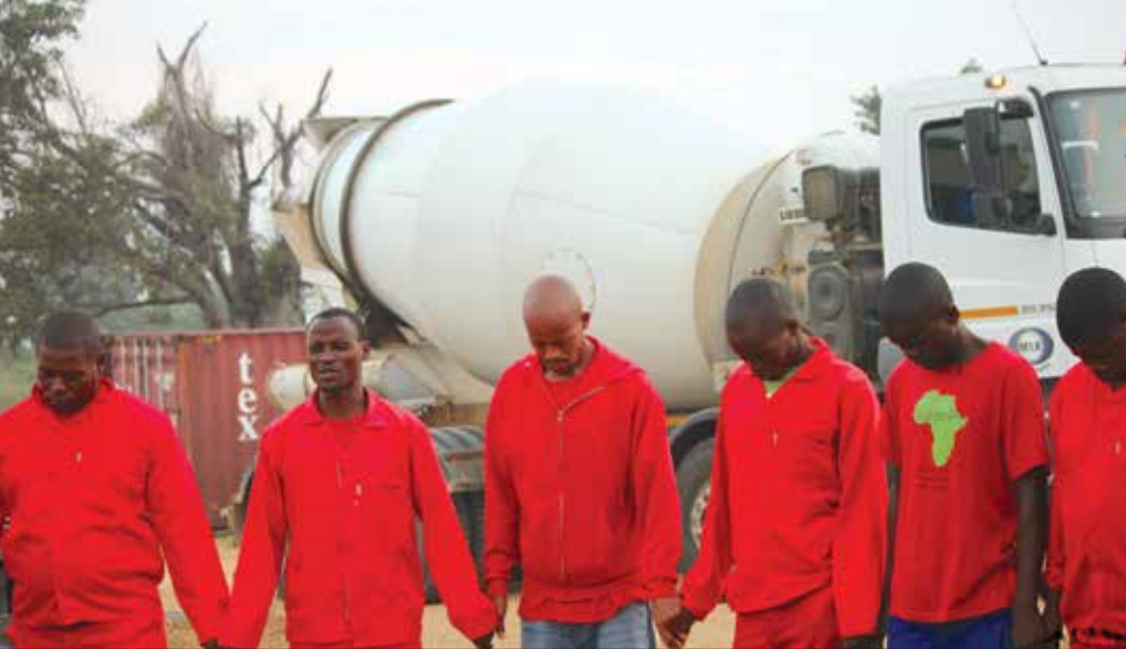
^ Prayer and praise first. As the first cement truck rolls onto the Miracle Campus, Thulani (second left) petitions Jesus for peace, calmness, safety, and joy on today's job site.
